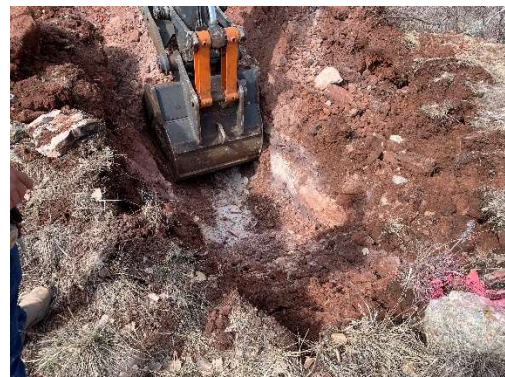
Figure 4 - Weathered rock that is diggable.
